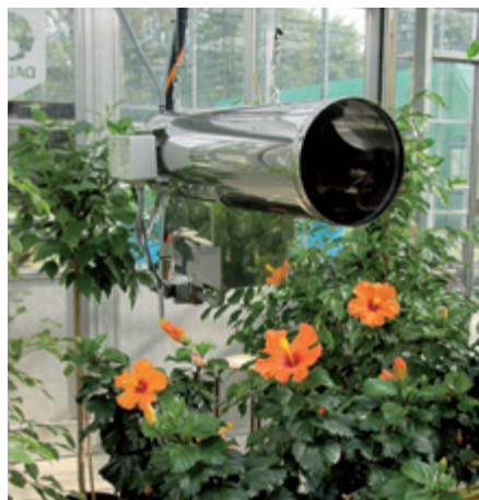
Era 33 33 kW gas burner with pilot flame for frost protection or for dosing of CO 2
