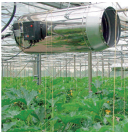
GP 95 95 kW gas burner
