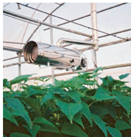
RGA 95 95 kW hot-air blower with chimney for diesel/kerosene
